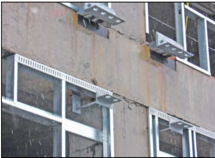
Figure 5: Panel Connection Points.
