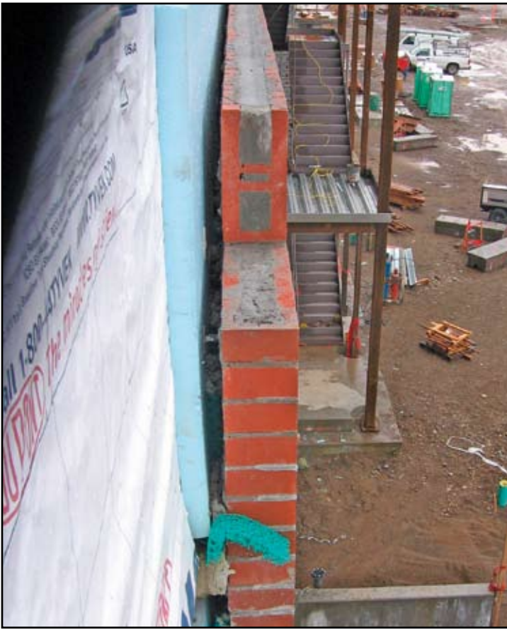
Figure 3: View of Wall Cavity.
