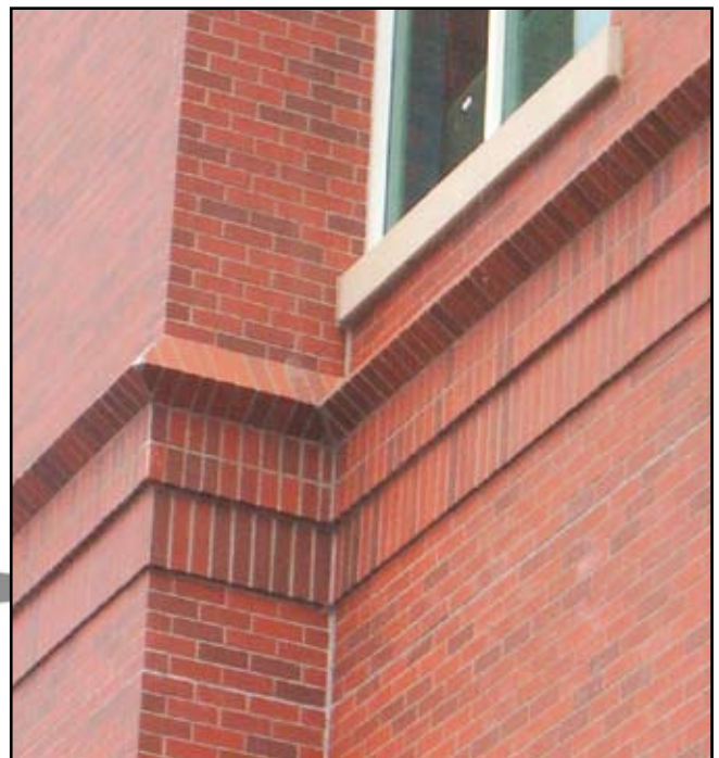
Figure 6: Closeup of Brick Feature Band.
