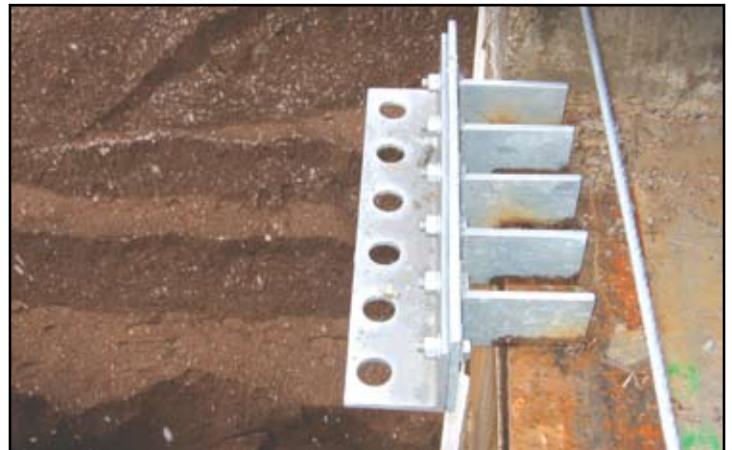
Figure 4: Typical Gravity Load Connector.
