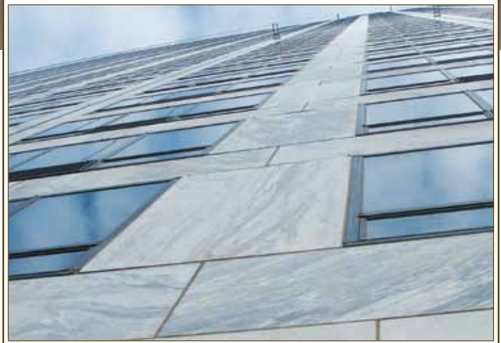
Figure 2: Overview of the metal-framed windows and marble panels.
