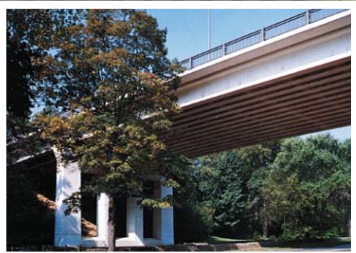
The original Walnut Lane Memorial Bridge in Philadelphia's Fairmount Park (1950). The main span is 160 ft (49 m) and the superstructure is about 50 ft (15 m) above Lincoln Drive.
