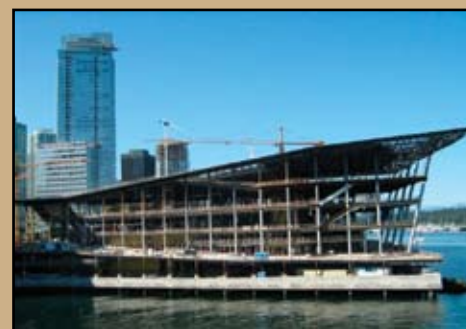
VCEC steel framed structure on marine deck.
