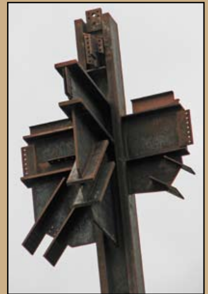
This gnarly column is a junction of full height wall trusses forming the primary framing system.
