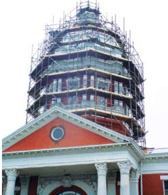
Scaffold around dome to facilitate repairs.
