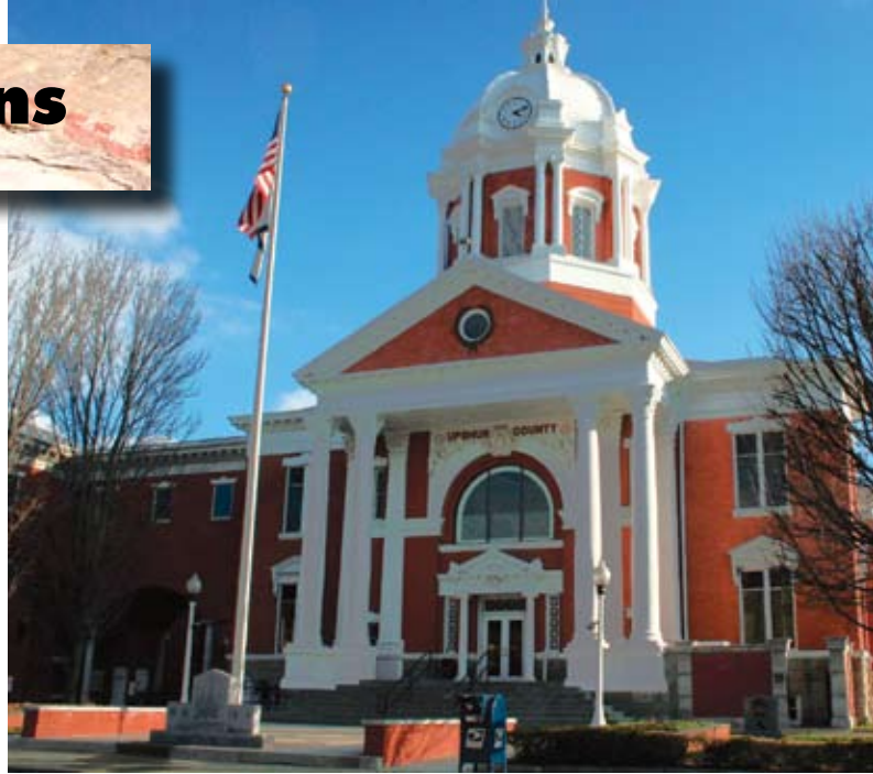
Restored dome and main entrance.
