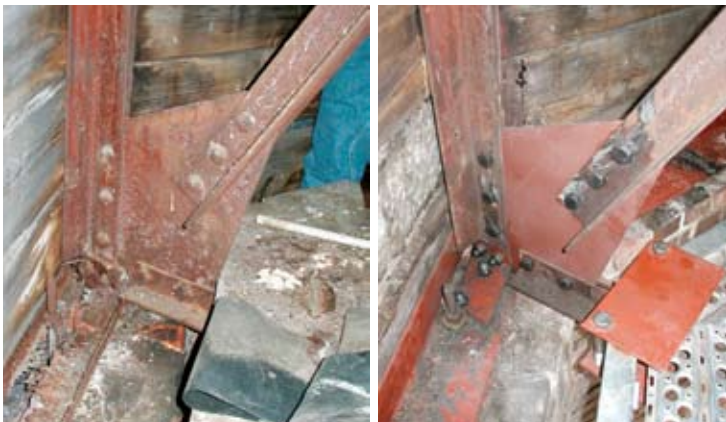
Left: Failed steel channel and riveted connection at truss. Right: Repaired connection at truss.
