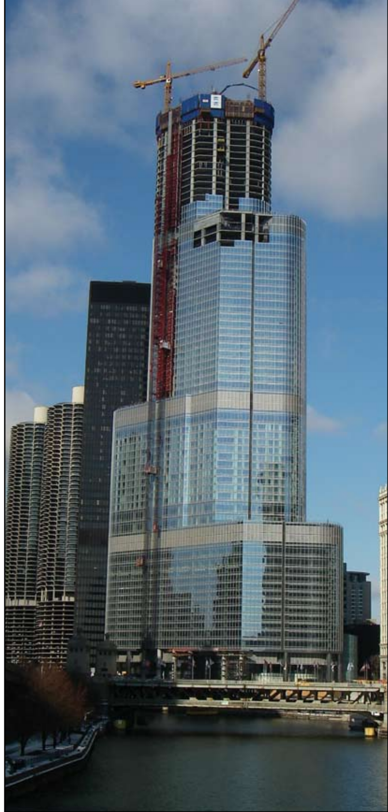
Construction progress – Spring 2008. Courtesy of Skidmore, Owings & Merrill LLP.
