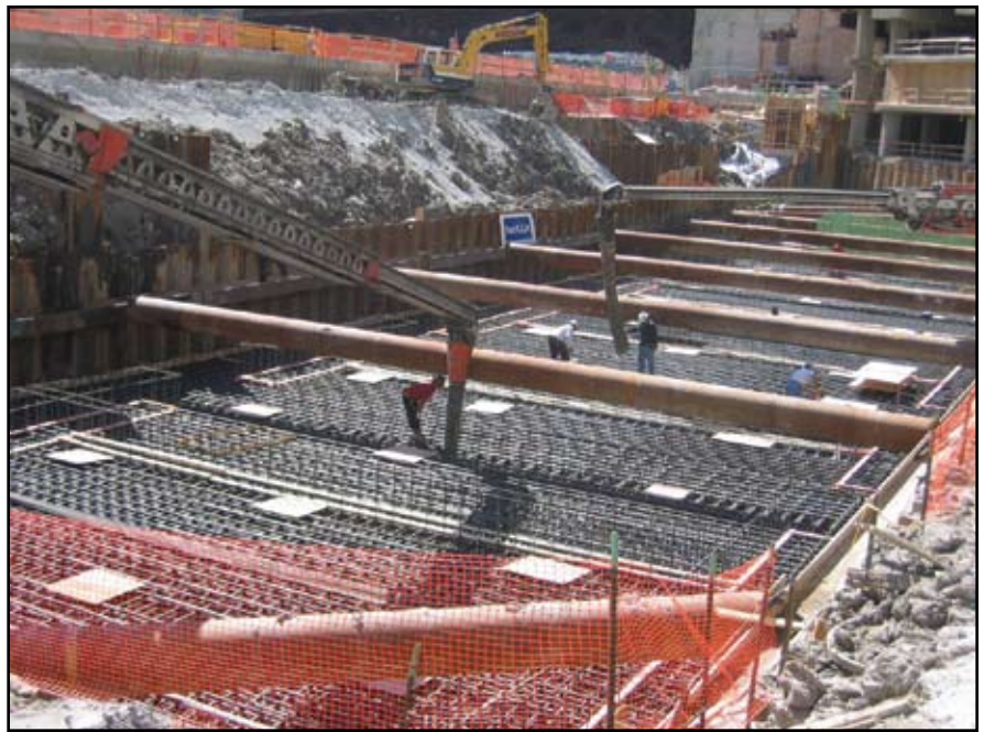
Mat foundation construction.
