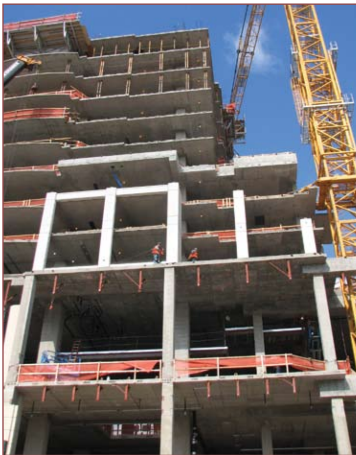
Concrete construction progress on one of the two residential towers.
