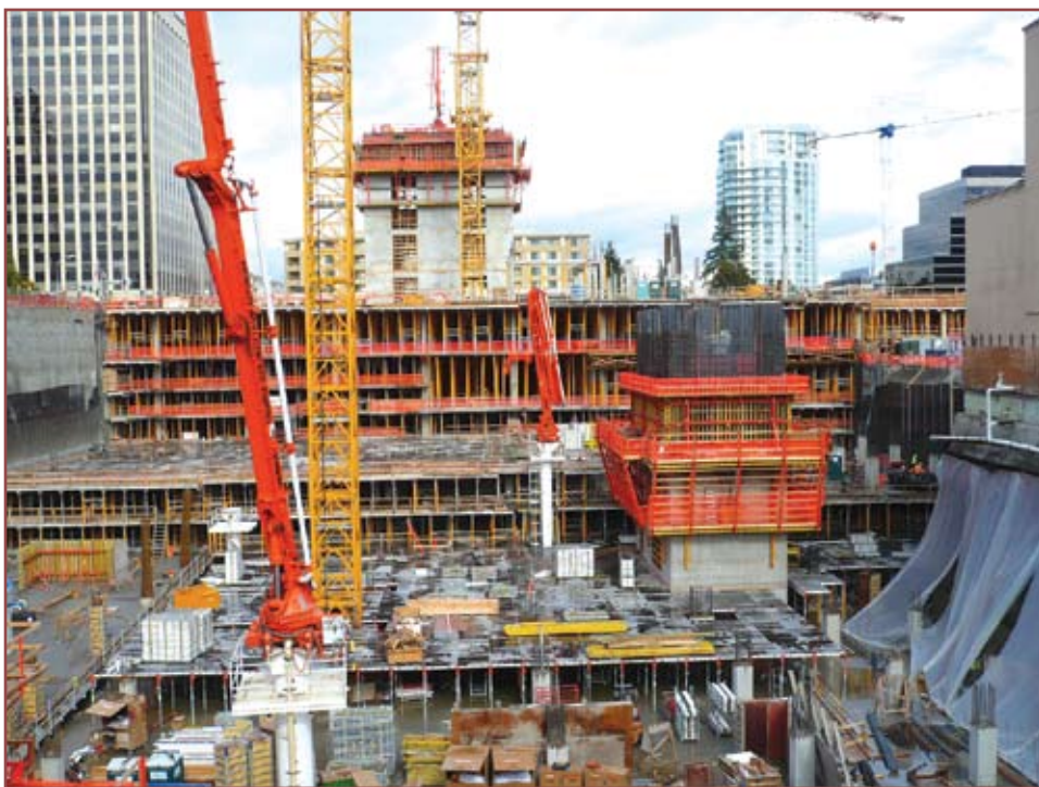
Early photo showing the various construction stages of the seven below-grade parking levels.
