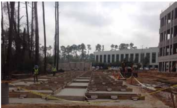
Phase 2 east side formed panels. Courtesy of E.E. Reed Construction, L.P.
