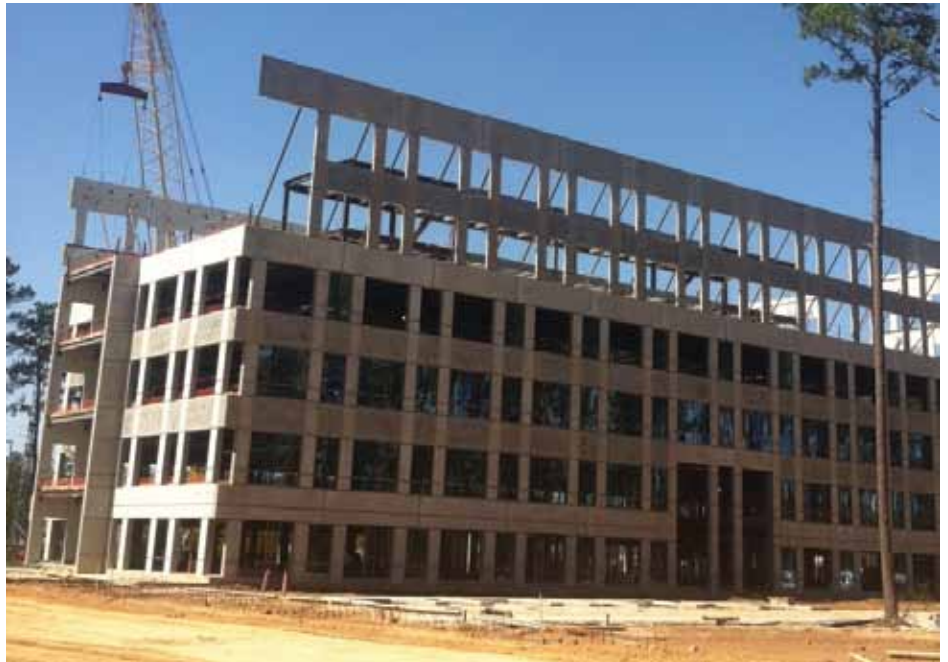
Overall building perspective looking at the east face as viewed from the parking garage. Courtesy of Big 4 Steel Services, L.P.
