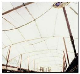
non-linear system, much of the load is carried by change of shape rather than change of stress. For instance, under snow loads, non-linear analyses show that the fabric hangs almost free between ridge cables, thereby taking on an optimal shape for carrying these loads in pure tension. In Denver, this sys-
