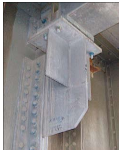
Figure 1: Installed seat bracket at Main Span.
