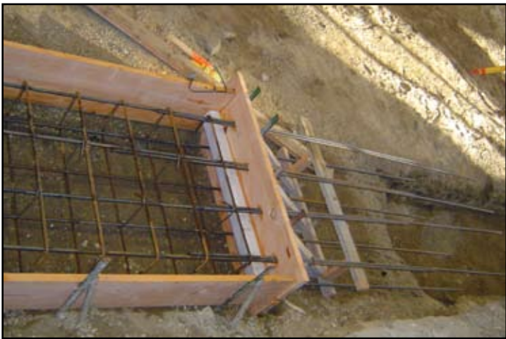
Figure 3: Footing reinforcing at step down to deep end of pool.
