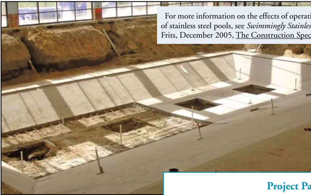
Figure 5: Foundations and partial slab at deep end of pool - showing diagonal shoring struts for building foundation.
