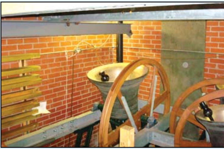
Figure 7: Bells in Up Position, Monorail System Above.
