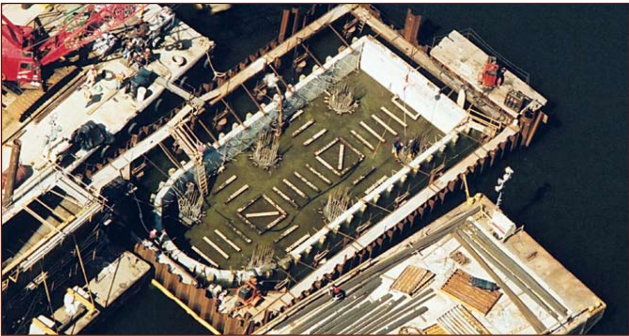
Figure 5: Precast Bathtub Nearly Complete. Courtesy of Morgan Kaolian/Aero, Inc.
