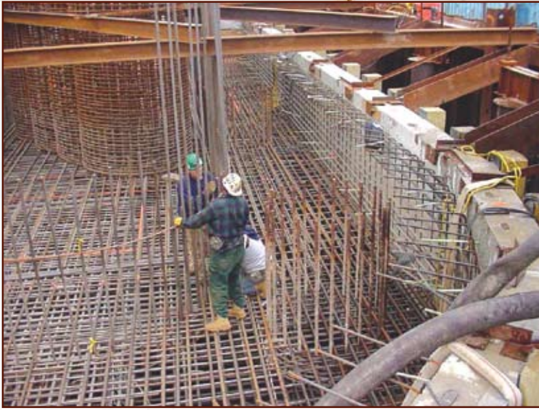
Figure 6: Rebar Installation Inside the Bathtub. Courtesy of William J. Frank, P.E.
