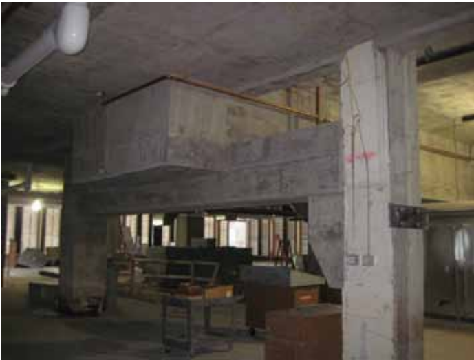
Figure 3: New concrete support beam below new swimming pool. Note the cast haunch and plate washer at back side of existing concrete column.
