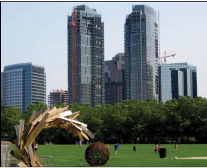
Bellevue Towers Project, Bellevue, WA. Courtesy of KPFF Consulting Engineers.
