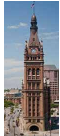
Milwaukee City Hall South Tower after construction. Courtesy of Eric Oxendorf.
