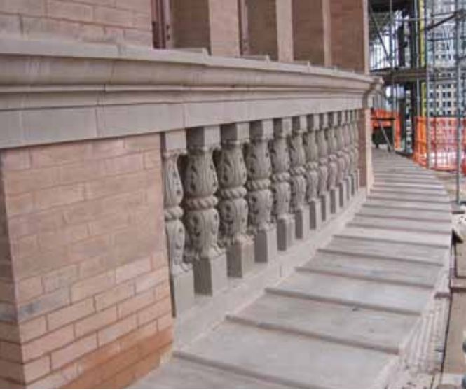
Figure 4: Typical terra cotta cladding with roll caps found throughout the structure.
