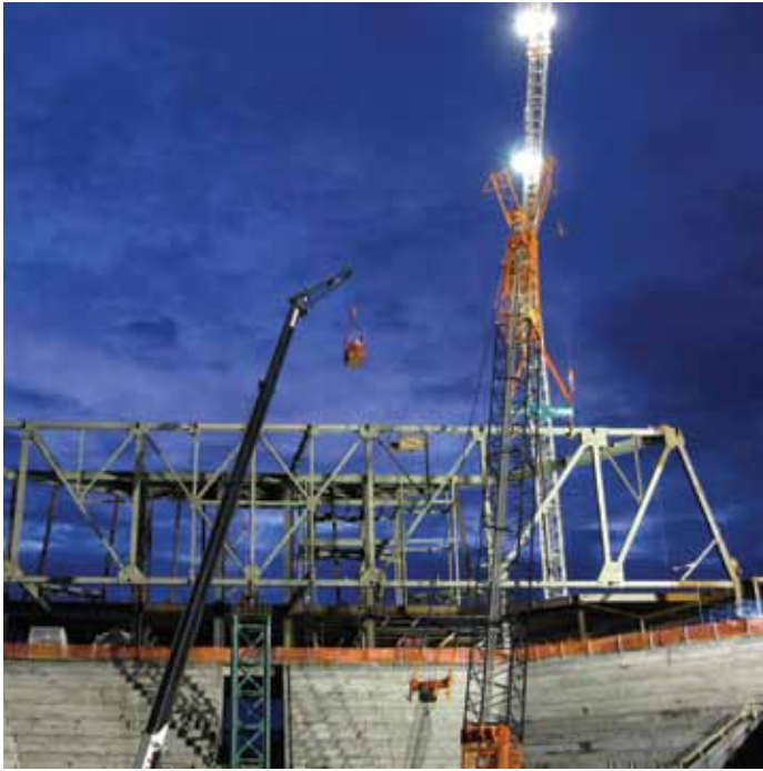
Figure 3: Roof truss erection. Courtesy of Hoffman Construction.
