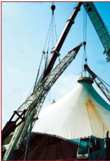
Removing the first mast (left) and inserting the top of the new mast (above).
