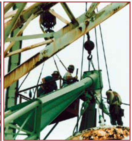
Removing the first mast (left) and inserting the top of the new mast (above).
