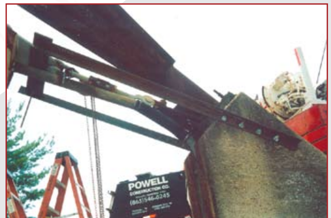
Temporary anchorage of cables.
