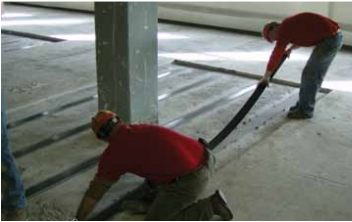
Carbon Fiber Install.
