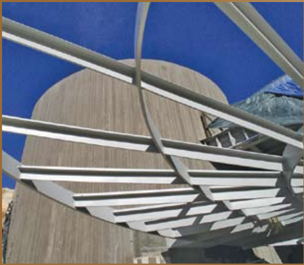
An elliptical steel awning, measuring 33 feet from front to back and cantilevering more than 27 feet past its forward supports, forms the centerpiece of the main entry to the exhibit building.
