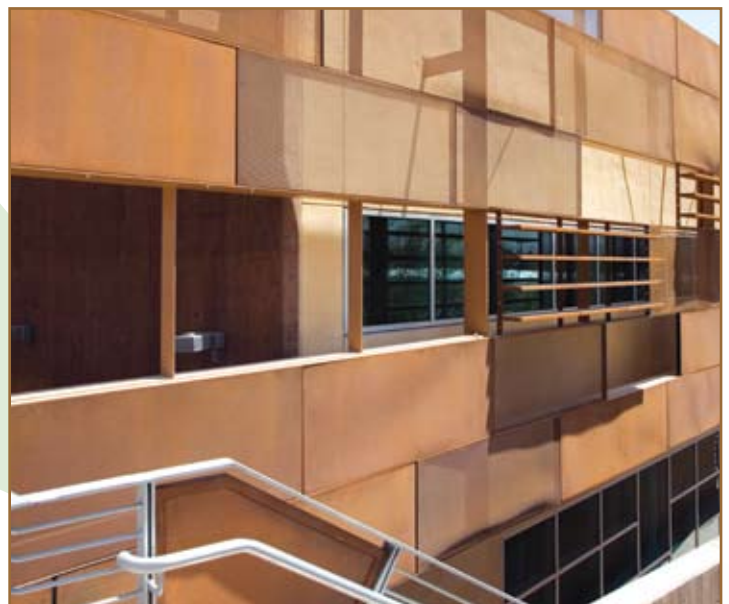
Exposed railings and interior screens required high level of detailing.
