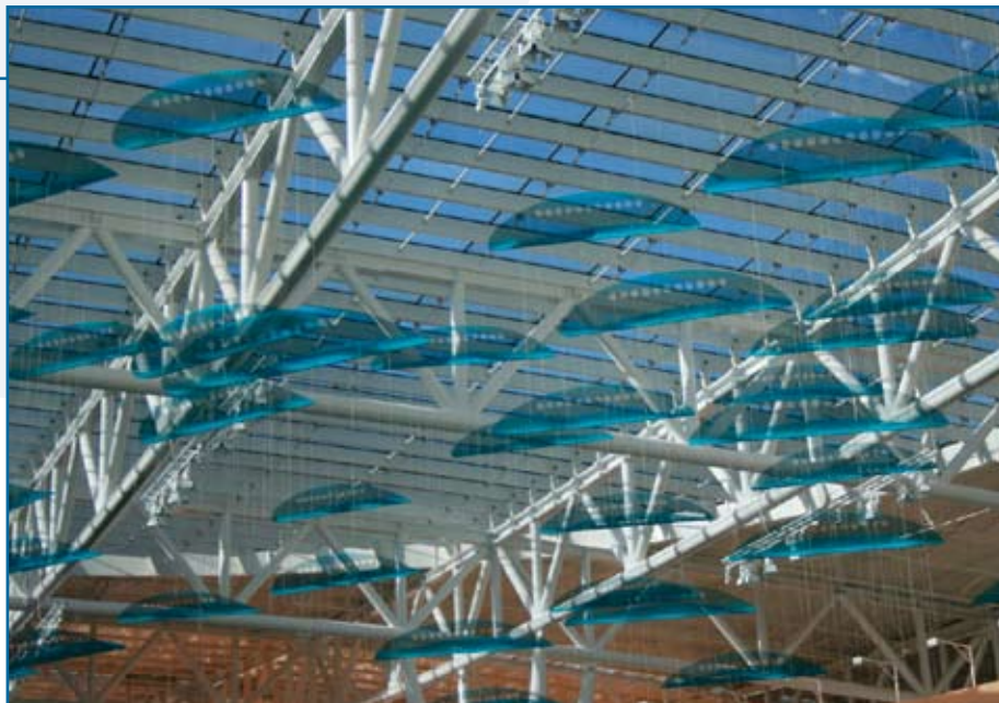
Skylight trusses support suspended artwork.
