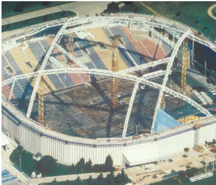
Figure 10: Unidome Construction Photo. Courtesy of DeNardis Associates.
