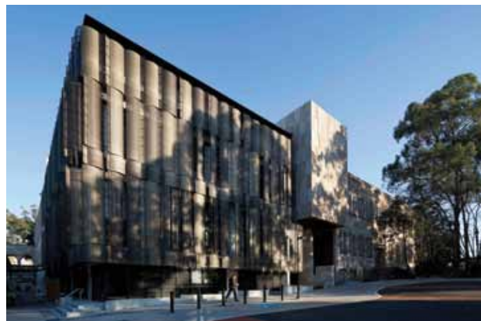
Figure 1: Completed Global Change Institute building. Courtesy of Angus Martin.
