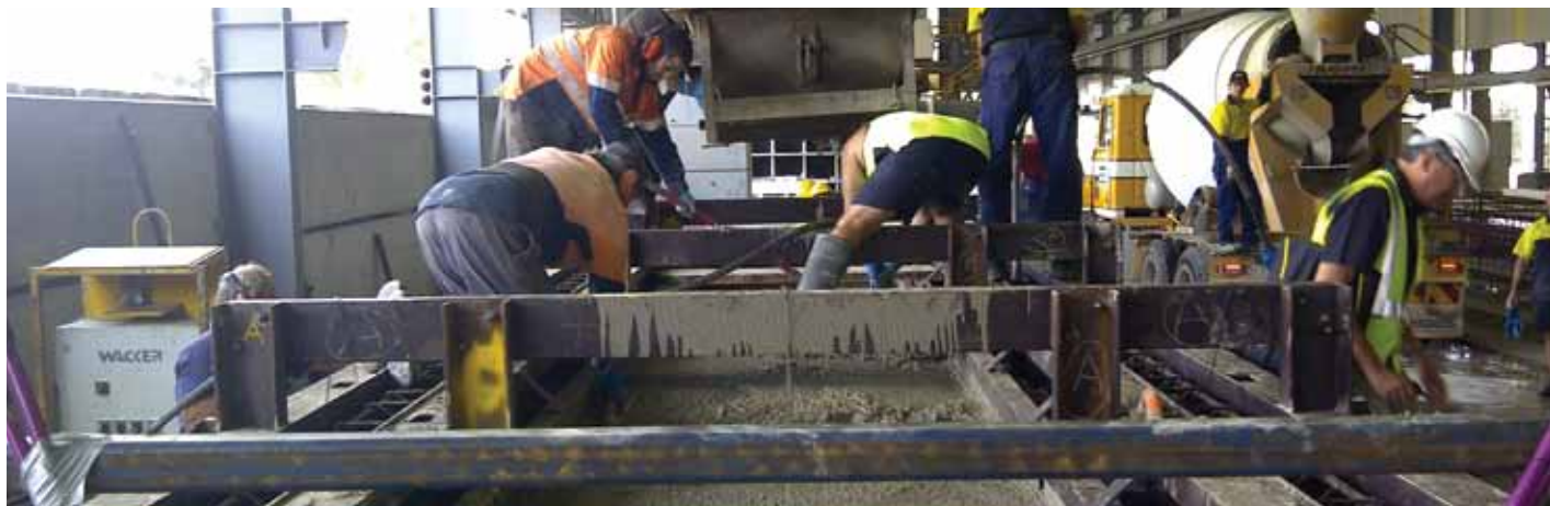
Concrete finishing in the precast factory. Courtesy of Wagners.
