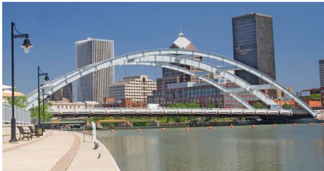
Figure 2: The New Frederick Douglass - Susan B. Anthony Memorial Bridge.
