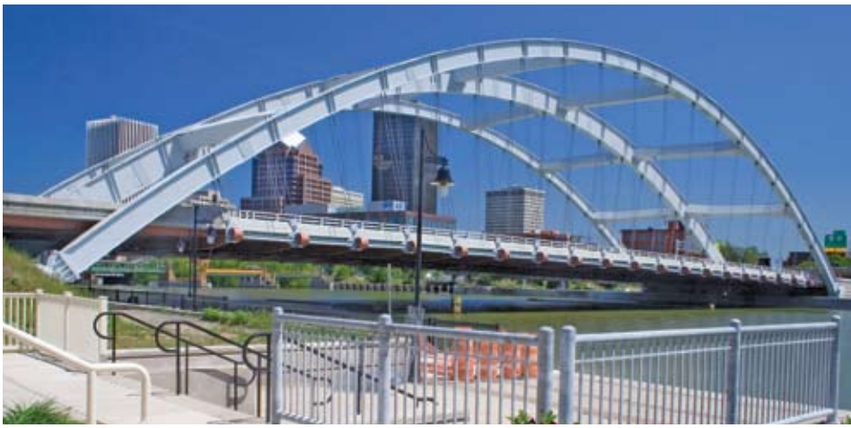
Figure 3: A Picturesque View of the Bridge from Corn Hill Landing.
