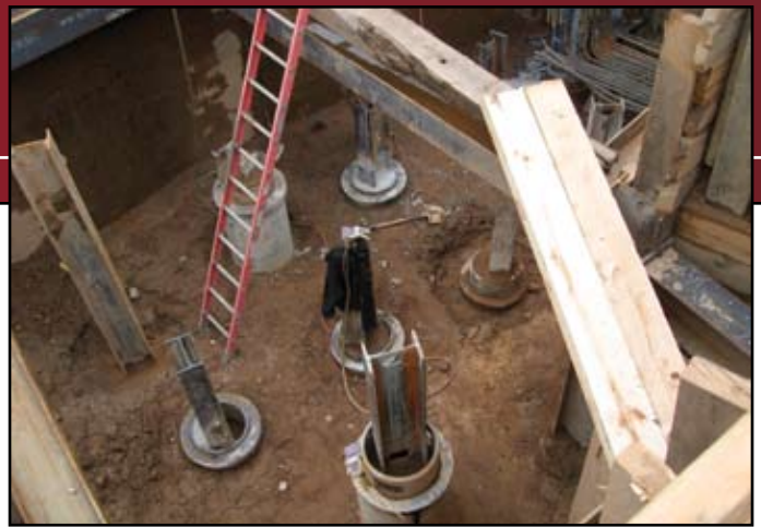
Drilled shaft foundations on the Schermerhorn House in Brooklyn, NY.
