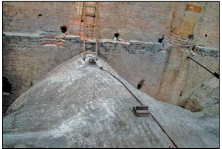
Figure 10: Brick Vault at Ulm Minster from above.
