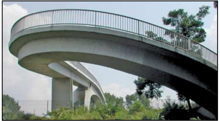
Figure 8: Cologne Concrete Bridge Cantilever.
