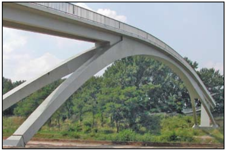
Figure 7: Cologne Concrete Bridge Span.
