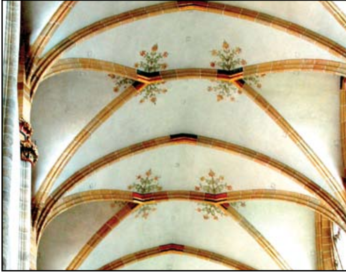
Figure 11: Ceiling Vault over Nave of Ulm Minster.
