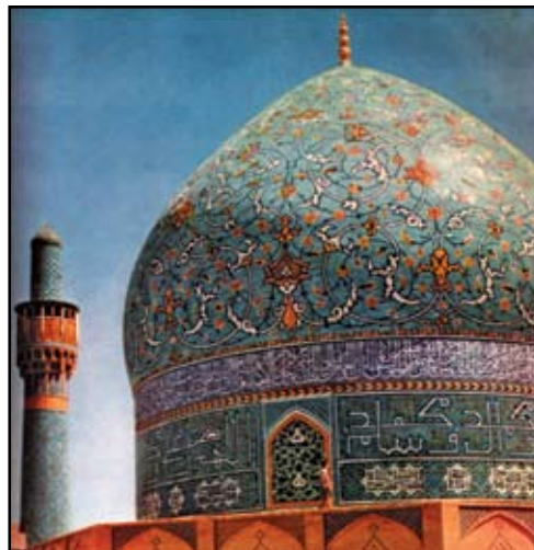
Figure 3: Tile covered brick ring dome of Royal Mosque in Isfahan, Iran.
