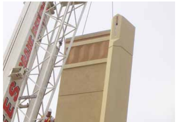
Figure 3: Prefinished corner element on pavilion building. Courtesy of Salamone Builders.
