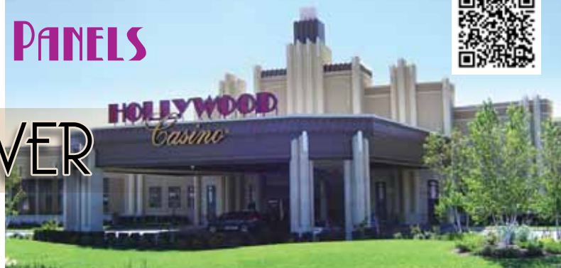
The new Hollywood Casino at Joliet, IL. Courtesy of National Prefab Systems, LLC.
