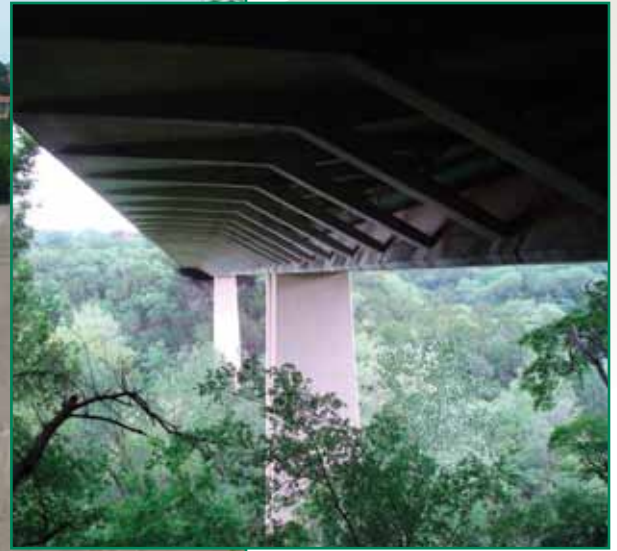
Figure 4: Underside of Barton Creek Bridge with Struts and Water Lines on Overhang and Twin Shaft Piers in the Distance.
