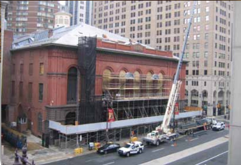
Construction underway at the Academy of Music.
