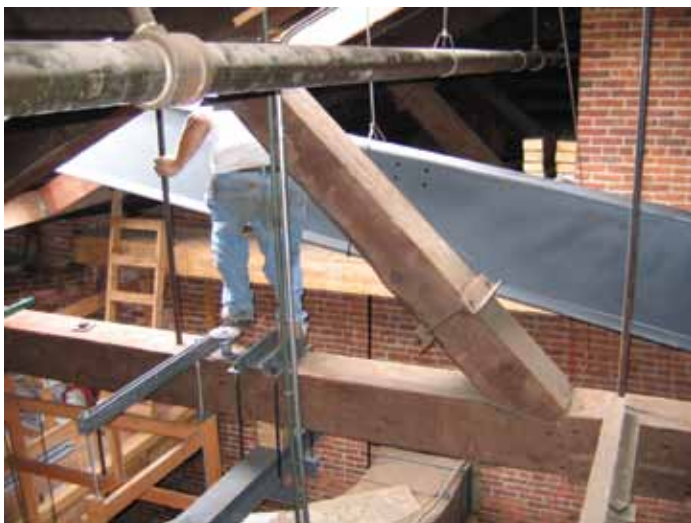
Attic view showing construction crew guiding new steel into place.
