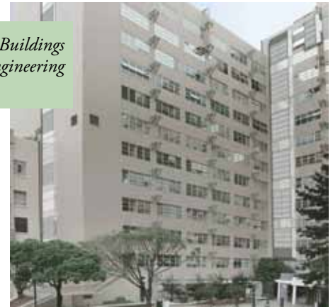
University of California, San Francisco MSB/Moffitt Separation Project.
