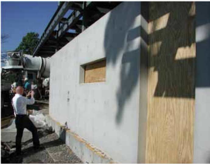
Architectural Concrete with knife edge corners and openings
