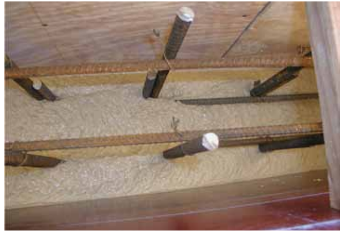
Architectural Concrete. SCC is pumped from the bottom in this wall.
