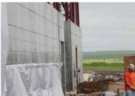
University of California, Merced, CA. Architectural Concrete Measured for Slump/Flow.
