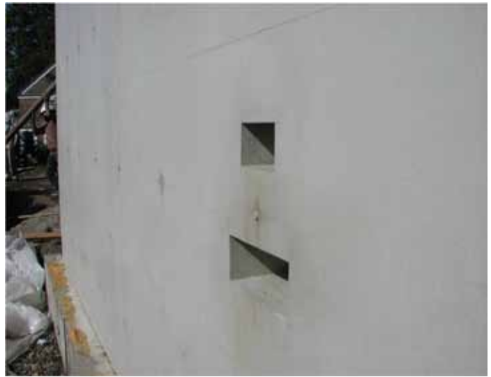
Architectural Concrete. Close up of knife edge openings.
