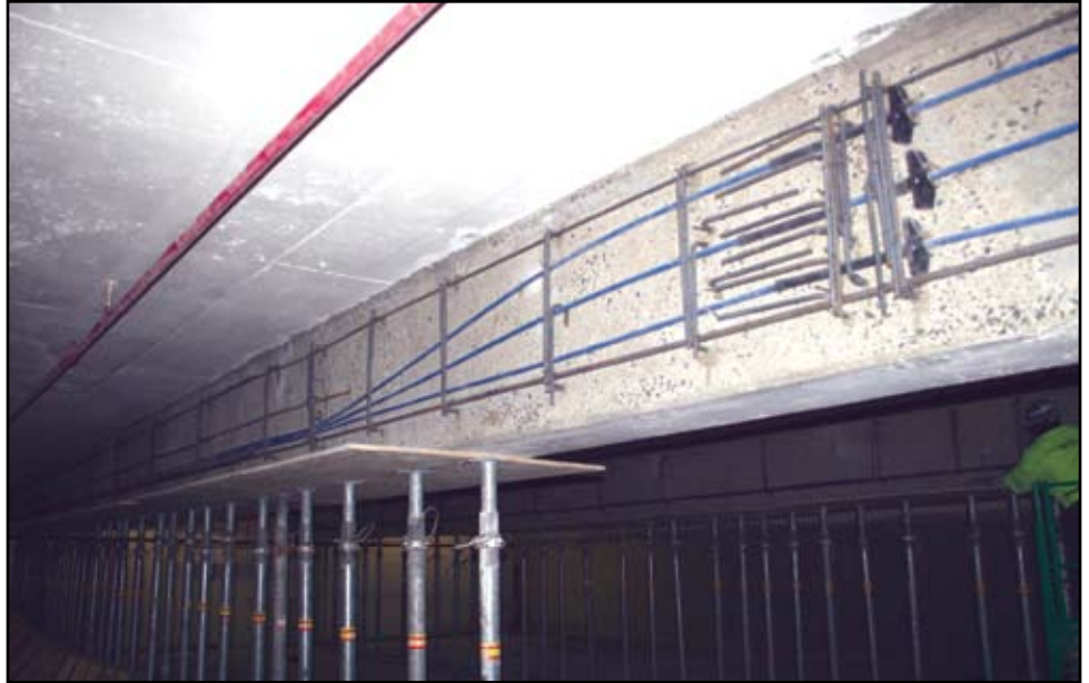
Installation of rebar, PT cables and anchors.
