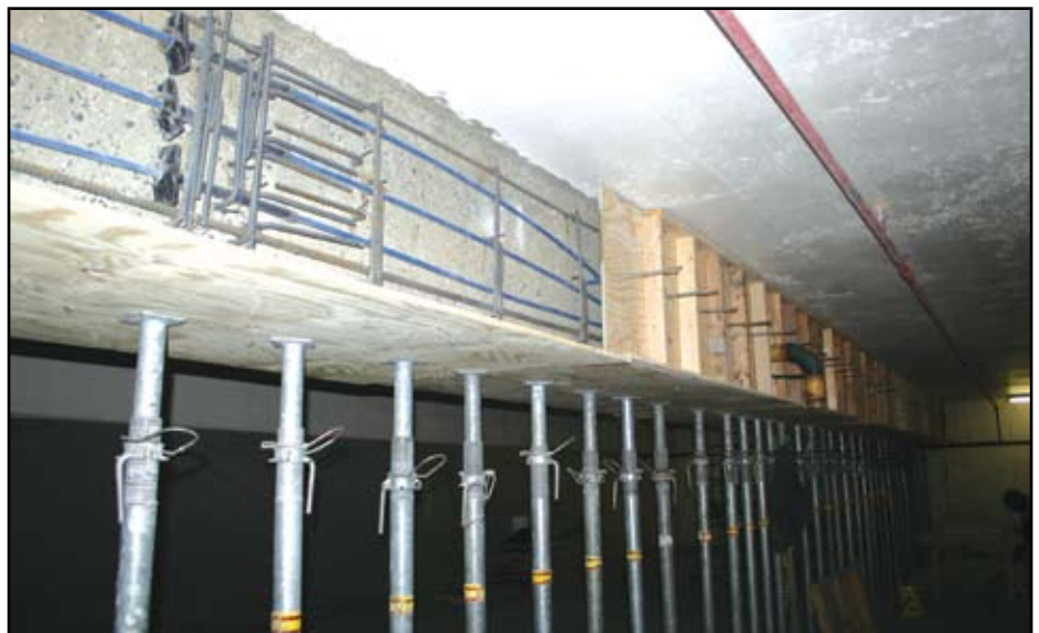
Installed rebar, PT cables, anchors and the formwork installation in progress.
