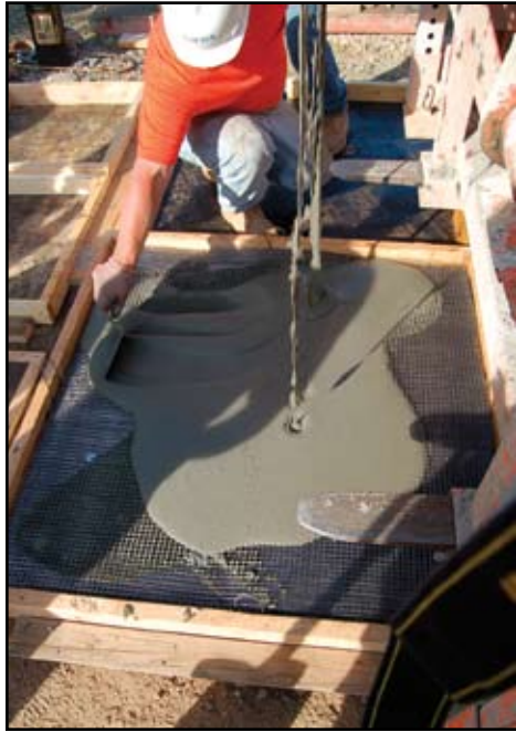
A highly flowable, self-consolidating cementitious slurry infiltrates the three-dimensional reinforcement mats, curing to an ultra-high strength mortar.
