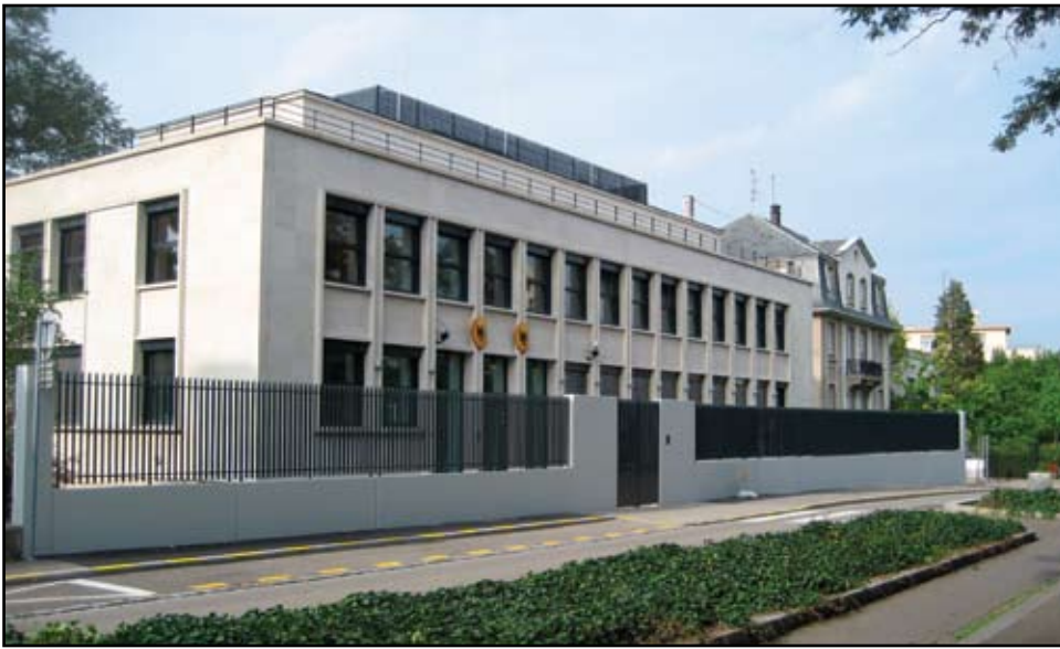
This consulate is a repurposed building that previously lacked blast resistance. The MRC blast-wall creates a secure perimeter between the building and the public street, and provides blast-protection both by deflecting shockwaves and stopping fragments from street-level car bombs or package bombs.
