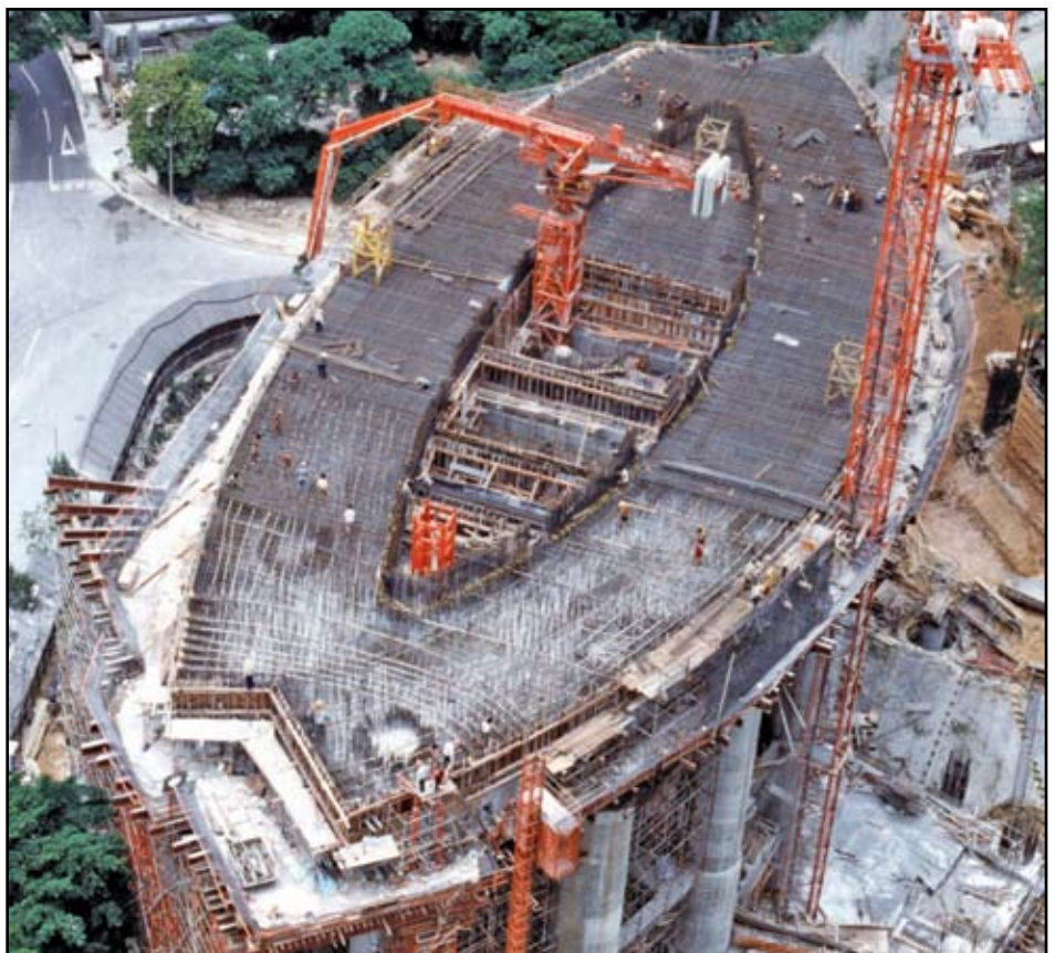
An aerial view of the transfer plate under construction.
