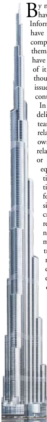
Rendering of the Burj Dubai Tower, Dubai, UAE Courtesy of Rowan Williams Davies and Irwin, Inc.
