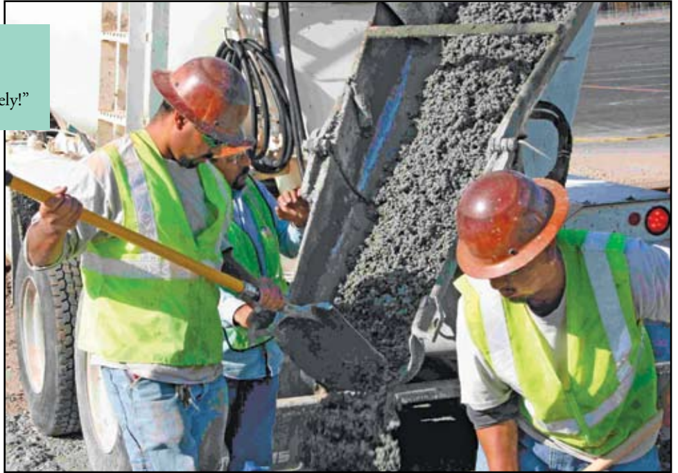
Fresh pervious concrete delivered to the jobsite.
