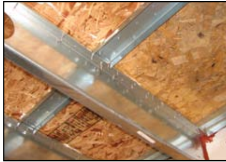
Figure 2: Engineered lumber (plywood or OSB) on CFSF.
