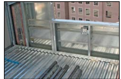
Figure 4: Pan deck and poured gypsum or concrete.
