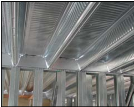
Figure 1: Composite poured concrete on Cold-Formed Steel Framing.
