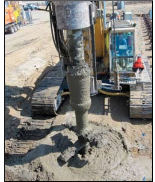
Wet soil mixing to stabilize soil and reduce lateral loads behind a sheet pile wall at the Port of Los Angeles Harbor. Courtesy of Justin Sharman.
