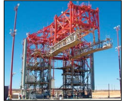
The Shuttle Mount/dismount structure resides at the west coast salt and sun environment. NASA selected inorganic zinc and polysiloxane to maintain the structure. Polysiloxane will retain color durability even in red. Courtesy of Coatings Pro Magazine.
