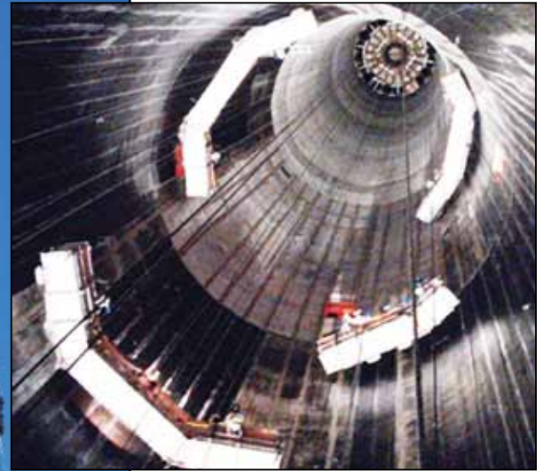
Figure 3: Application of FRP on Exterior (Left) and Interior (Above) of Plum Point Chimney.
