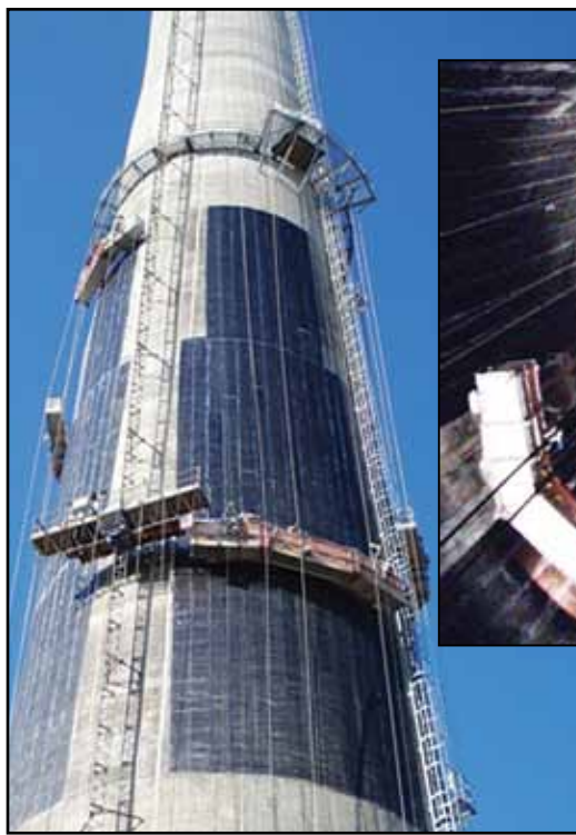
Figure 3: Application of FRP on Exterior (Left) and Interior (Above) of Plum Point Chimney.
