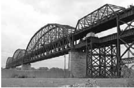
Municipal Bridge, now called the MacArthur Bridge.
