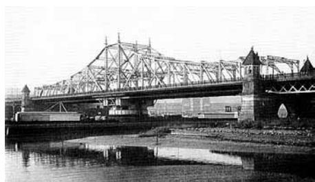
Thames River Bridge.
