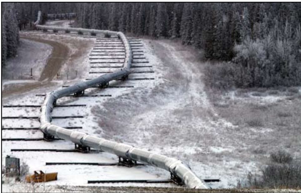
Trans-Atlantic Oil Pipeline, Alaska. Courtesy of USGS.
