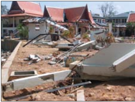
Column failure of a reinforced concrete frame.
