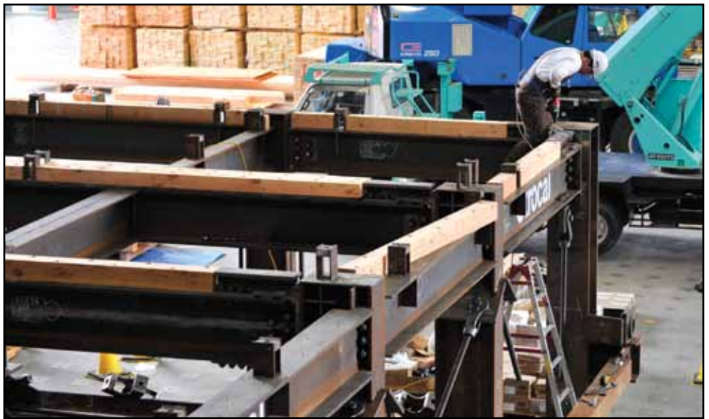
Figure 2: Wood Nailers Being Installed on Steel Frame.
