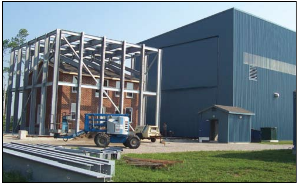
The 3 Little Pigs facility at the London airport site. The cover building has been rolled back to show the test house inside the steel reaction frame.
