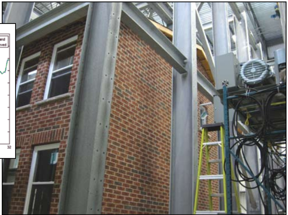
The first test house will undergo a series of tests over a 2 year period and will be ultimately tested to destruction. Tests can be repeated precisely for the evaluation of incremental building improvements.
