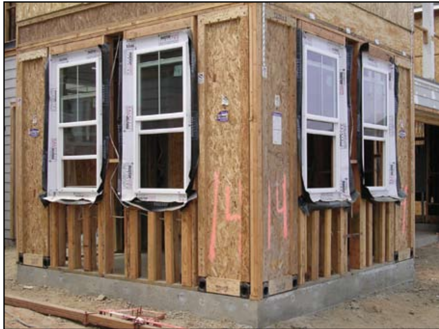
Figure 1: Prefabricated Shear Panels in Application.
