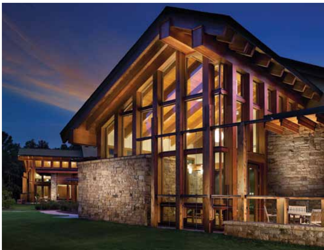
Sustainability goals for the Willson Hospice House in Albany, Georgia were achieved with the help of wood structural and finish materials, as well as timber reclaimed from a local cotton mill. Architect – Perkins+Will; structural engineer – Uzun & Case; photo – Jim Roof.
