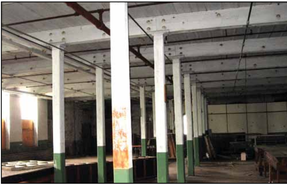
3-Span Continuous Wood Beams.
