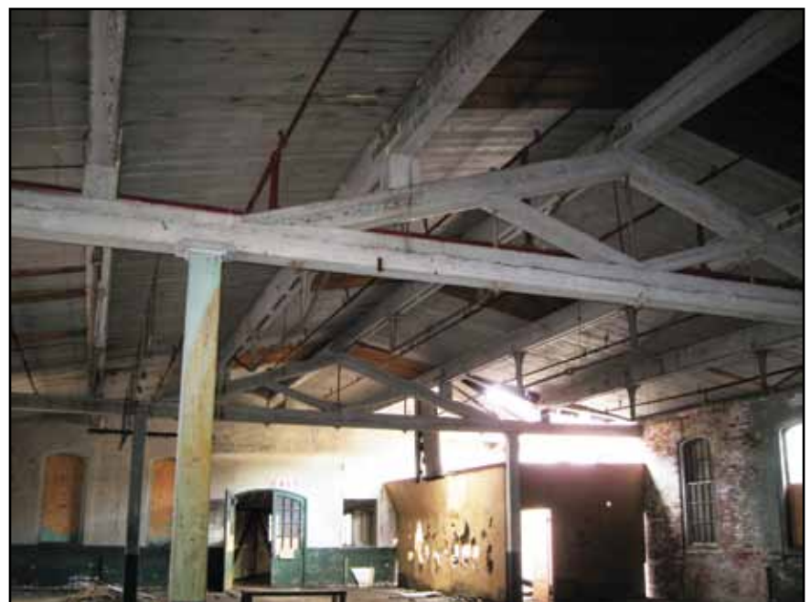
Queen Post Truss Spanning Between Gable Truss.
