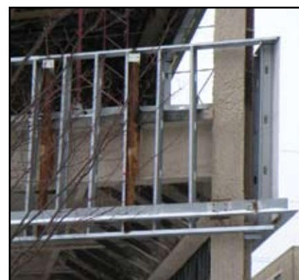
Typical Shelf Angle in Brick Veneer Construction.
