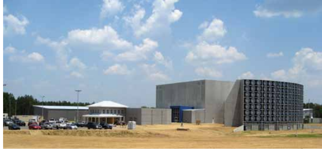
An overall view of the IBHS Test chamber and office building. Courtesy WALTER P MOORE.
