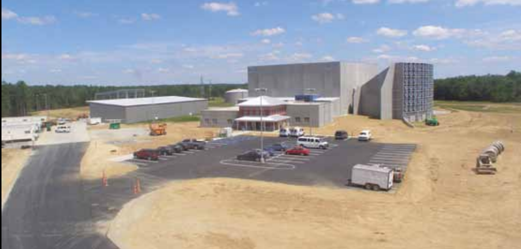
An overall view of the IBHS Research Facility. Courtesy of IBHS.
